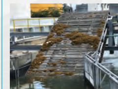
Development and setup of a mechanical protection system against gulfweed inlet, in the Barahona Power Plant Capacitor
